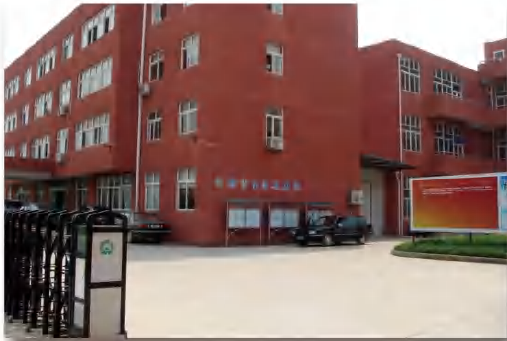
厂房大楼 Factory building
